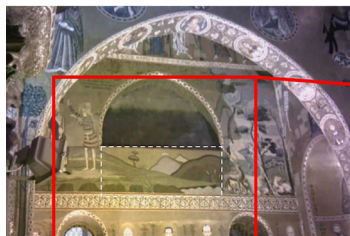
Figure 11 Infrared observation performed on the North wall of the North transept of the Cappella Palatina in Palermo, showing the presence of a walled-up portion of the window. Graphic: TecnoArt.
